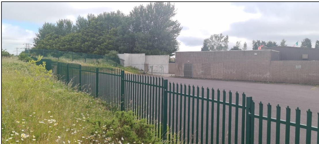
Photo 12.9: Delaneys Clubhouse presenting a blank elevation towards the site boundary.
