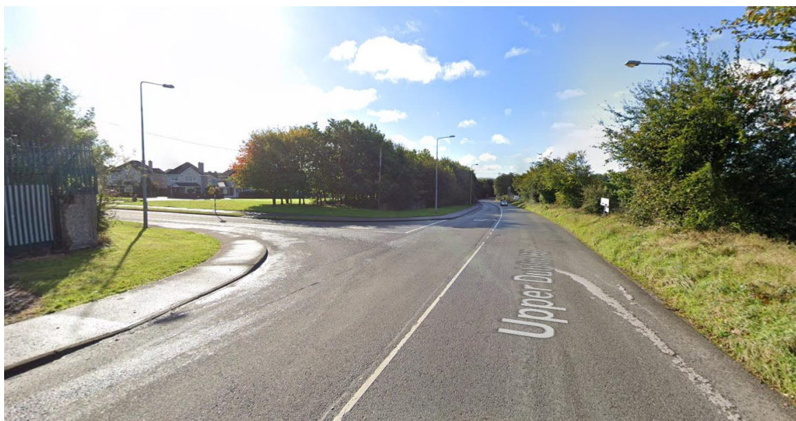
Figure 7.18: Upper Dublin Hill/ Lower Dublin Hill Junction
