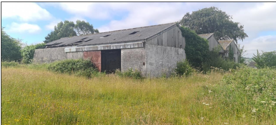
Photo 12.22: Disused workshop on the western side of the development site due for demolition.
